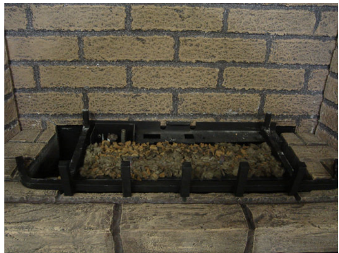
Figure 54 - Rock wool placement
